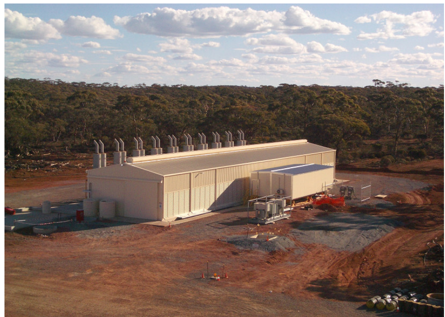
Figure 7. Higginsville diesel power station
