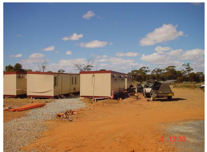
Figure 4: Construction of new rooms for camp expansion.
