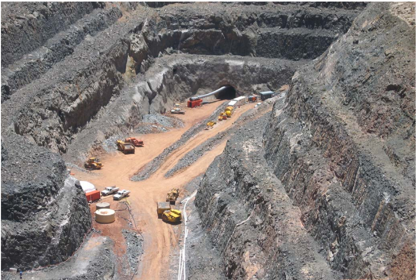
Figure 1: Commencement of underground development at Trident.
