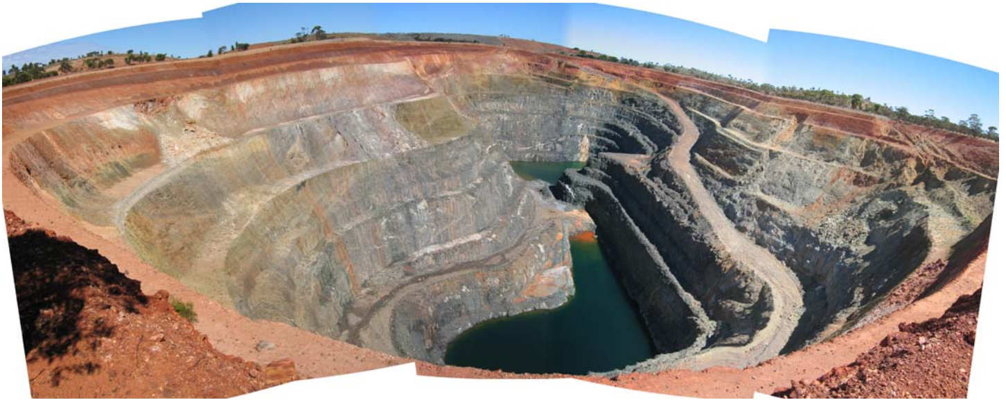
Figure 1: Photo mosaic looking south at the Poseidon South open pit. The water in the foreground (north end of the pit) is currently being pumped into the sub-pit in the background of the photo (south end of the pit) to allow refurbishment of the underground workings prior to Avoca commencing development to the Trident deposit.
