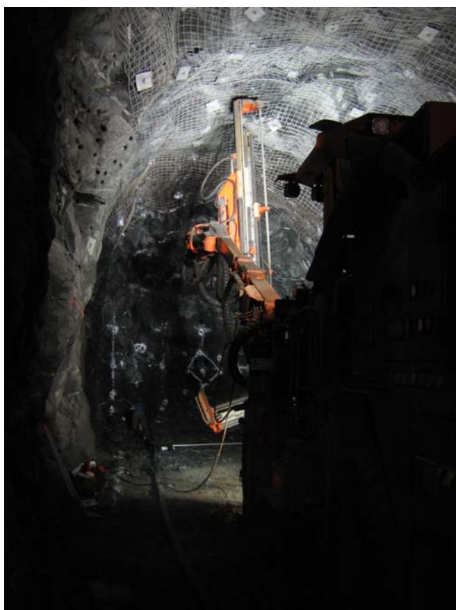
Figure 2: Ongoing rehabilitation work of the Poseidon South Decline
